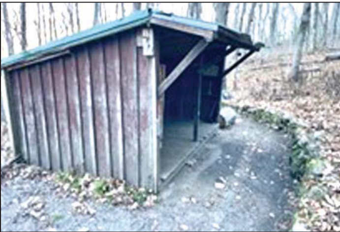
Rock Gap Shelter before renovation
