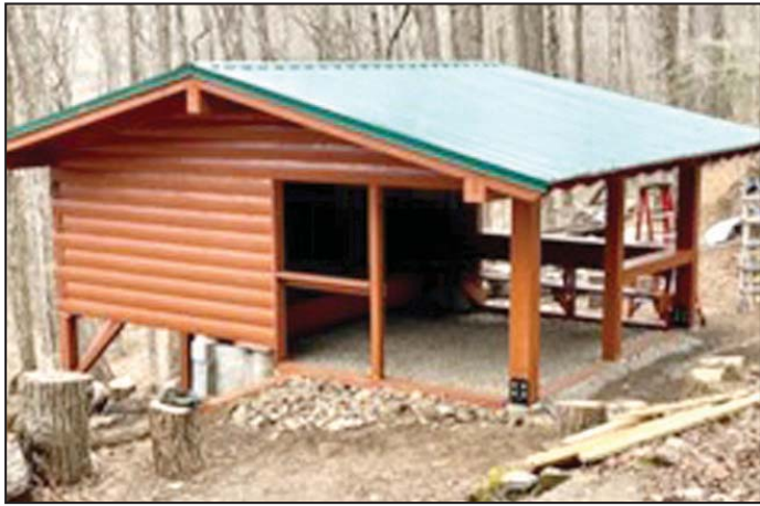
Renovation of Rock Gap Shelter February 2023
